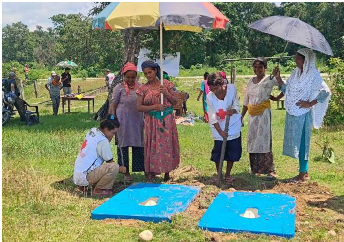
Nepal Red Cross Society volunteers and local people mobilized to support the community to build temporary latrines in an evacuation centre. (Photo: NRCS)
