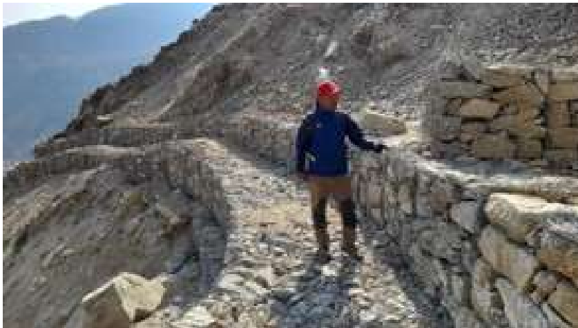
Figure 6: Retaining walls to protect the communities
