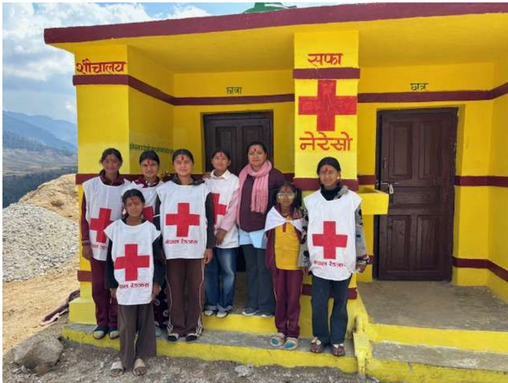
Figure 1: Gender friendly toilets for a school with the Red cross Youth cycle
