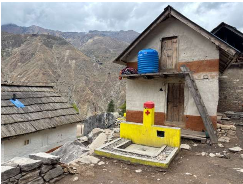
Figure 2: construction of a water scheme with a distribution system that gives each household access to safe drinking water
